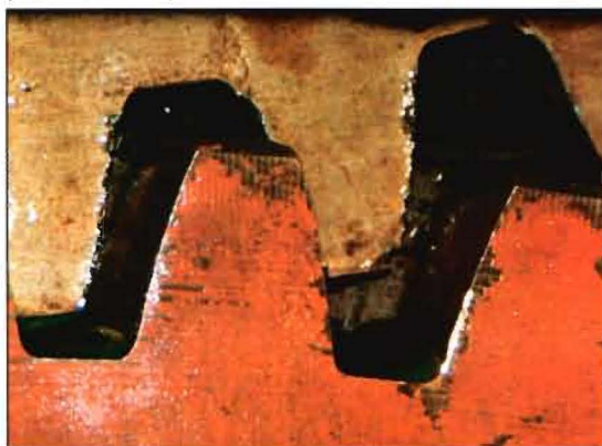
FIGURE 1: Misalignment is one of the easiest problems to spot.
